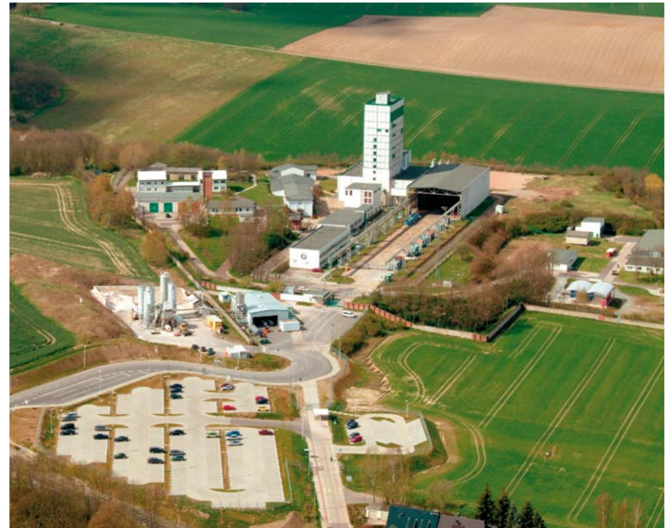
Abb. 1: Schachtanlage Bartensleben / surface facilities of the Bartensleben mine (Foto: BfS)
