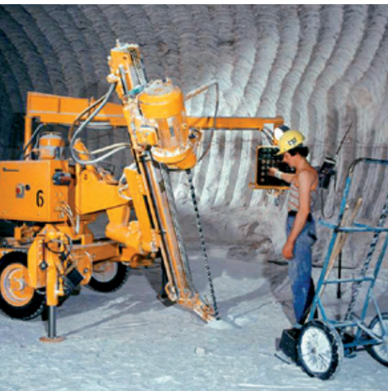
Abb. 2: Korfmann – Strossenbohrwagen / Bench drilling jumbo – Korfmann
