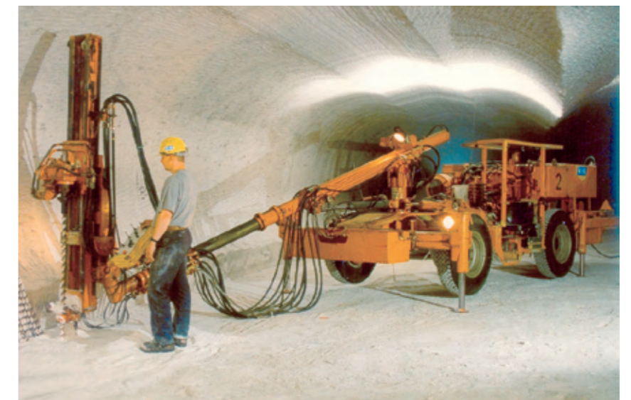
Abb. 4: Schell – Strossenbohrwagen / Bench drilling jumbo – Schell
