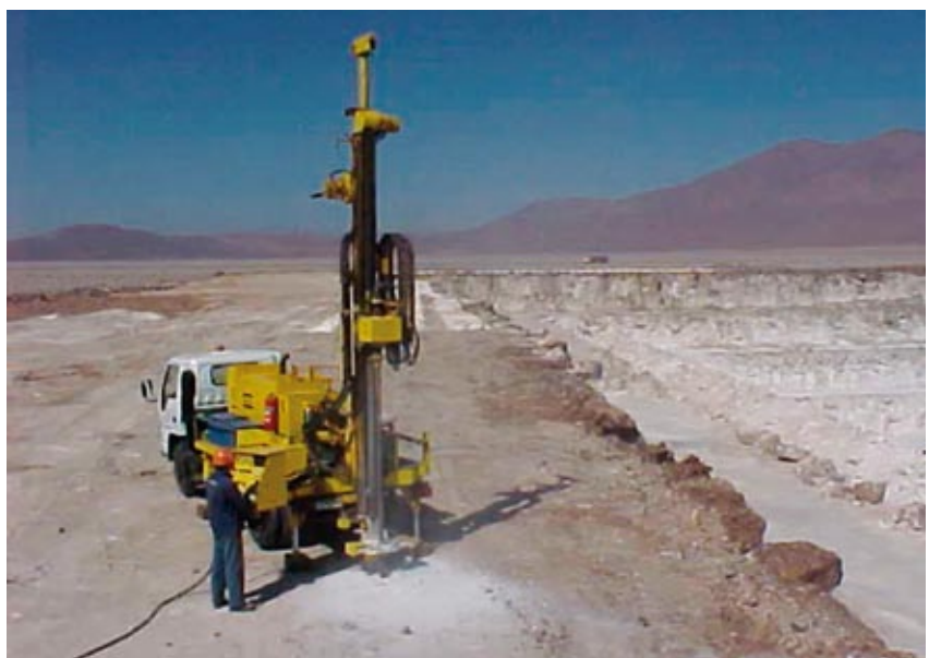
Abb. 7: Explorationsbohranlage. Foto: SPL / Exploration drilling machine. Photo: SPL
