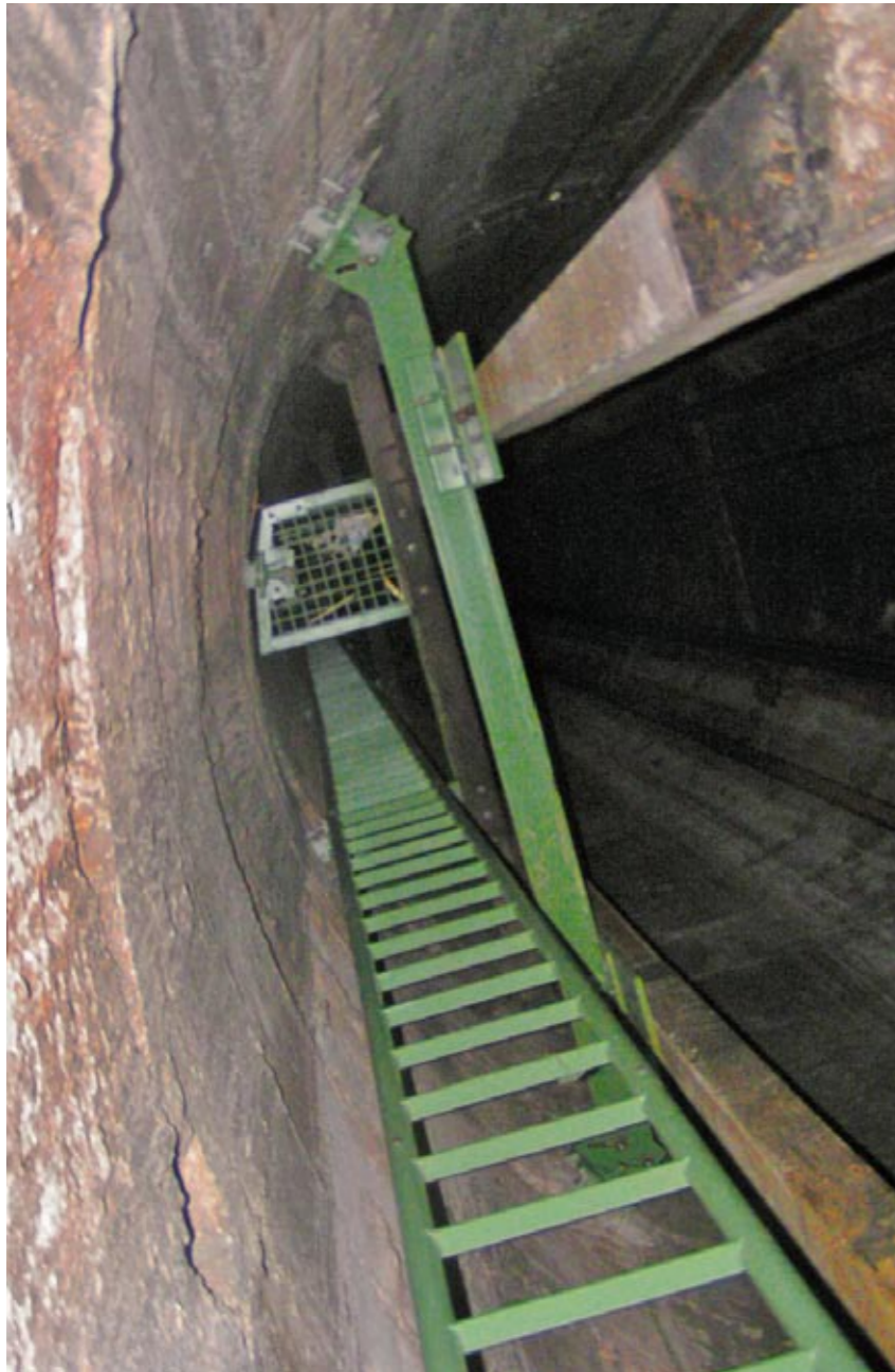
Abb. 5: Neues Fahrtentrum / New ladder compartment
