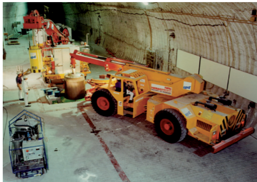
Abb. 11: Demonstrationseinlagerung hochradioaktiver Versuchsquellen (Kalterprobung) | Demonstration of the disposal of high-active waste (testing with dummies)
